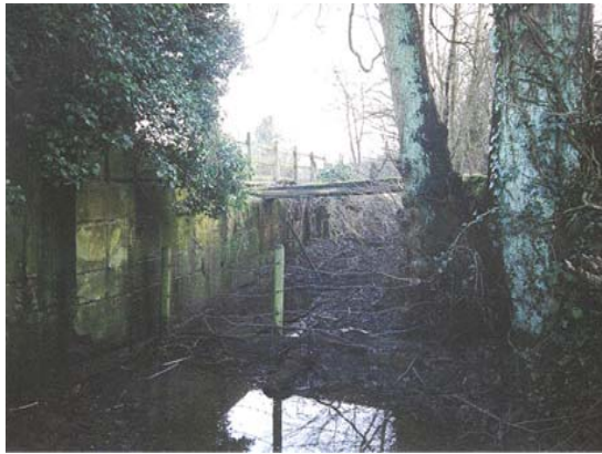
Churnet Flood Lock off Crumpwood Weir
